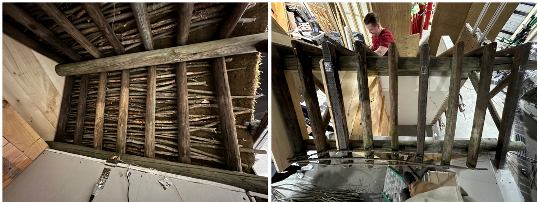
(a) Lab scale finished roof from below
