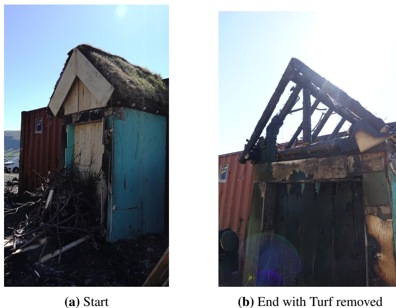
Figure 22: Photos of door scale Burn 5
