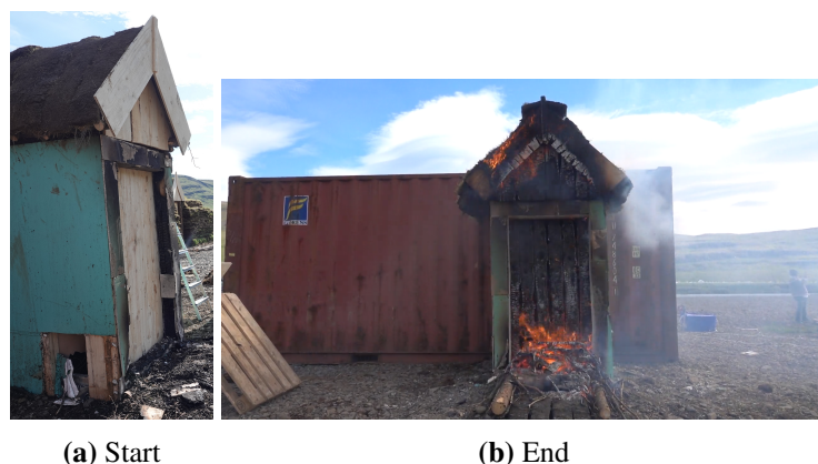
Figure 21: Photos of door scale Burn 4
